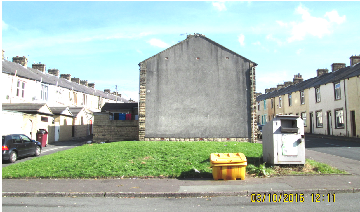
the site viewed from Burleigh Street
