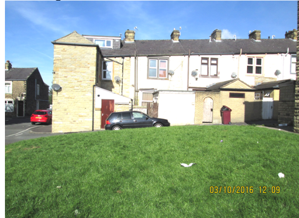
looking towards rear of March St houses
